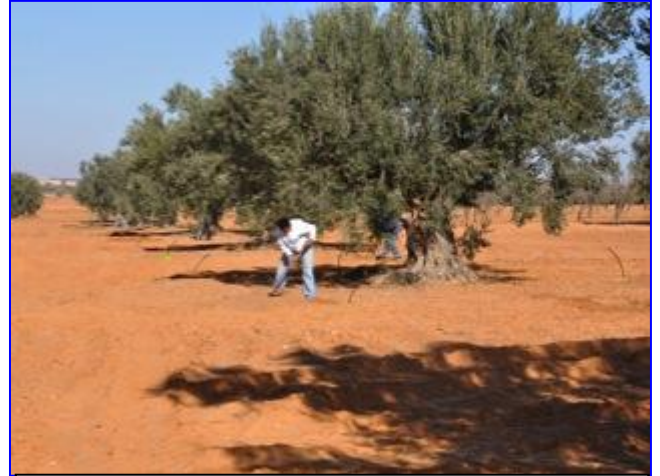
Installation of diffusers for olive trees in a private plantation in Sfax, South of Tunisia
