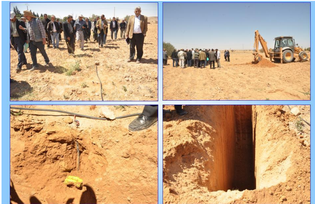
Trial water injection in the deep soil layer using the buried diffuser. One diffuser has injected 10 000 liters during 1250 hours nonstop (52 days). To see the underground distribution of the 10000 liters , a trench has been dug 3 meters deep and 10 meters long. This trench showed that the wetted soil under the diffuser (humidified bulb) has 2 meters deep and 6 meters diameter
